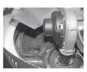
Photo 44 shows heater with collector cover removed allowing Step 8. access to anode rods and flue baffles.
